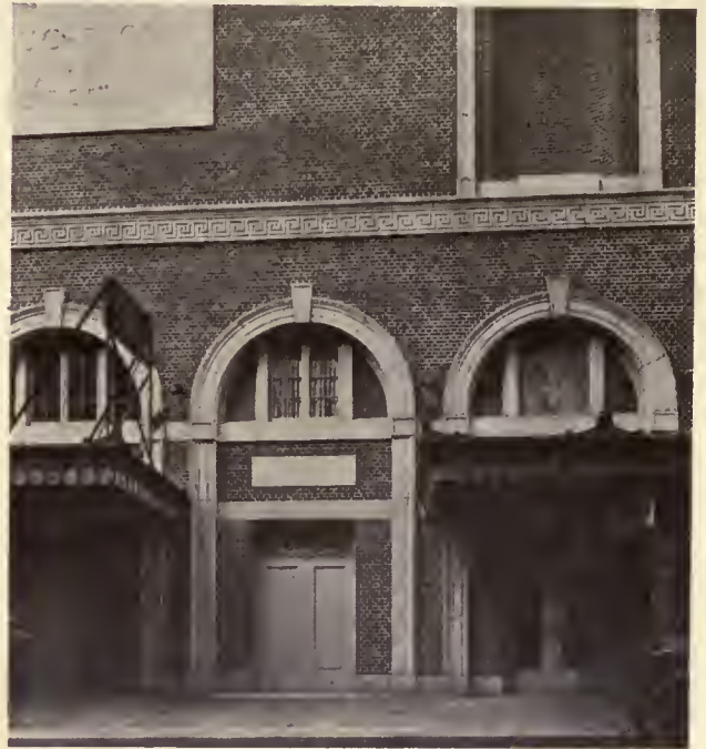
ENTRANCE DETAIL THE TOWN HALL, NEW YORK CITY McKIM, MEAD & WHITE, ARCHITECTS
